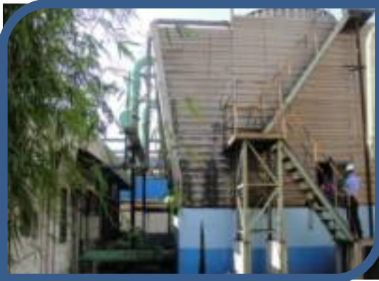
PEKERJAAN COOLING TOWER PT.ISPATINDO
