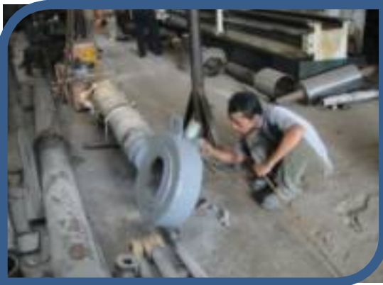
REPAIR ROD KAPAL PT.DOK
