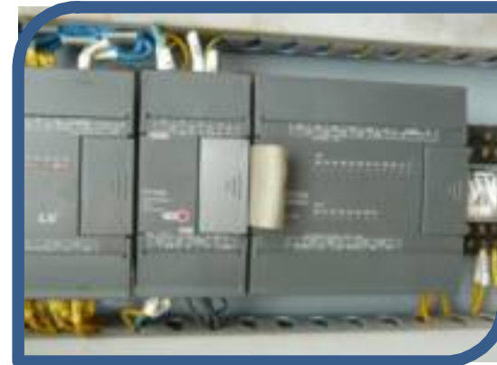
REPAIR INVENTER CRANE 50 T PT.DOK
