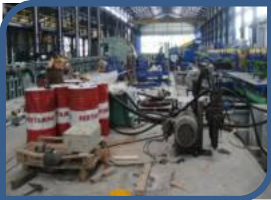
OIL FLUSHING PT. BHIRAWA STEEL
