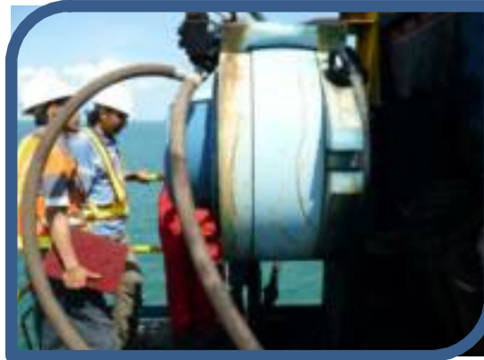
REPAIR HYDRAULIC MOTOR PT.DOK
